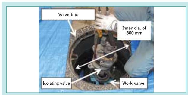
Fig. 11 Replacement Work Inside Valve Box
