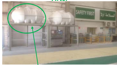
KSACO Added 3,000 Ltr. Drinking Water Tank to Reduce Water Waste, Time Consuming and Cost.
