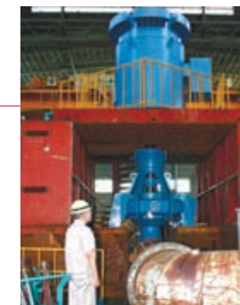
Trial operation of pump
