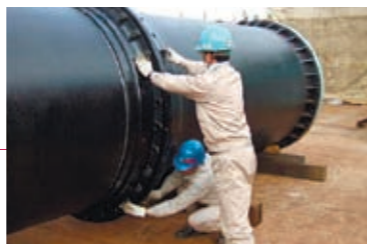
KUBOTA's new joints were adopted by the U.A.E. for their 47-km pipeline composed of huge 1,600-mm-diameter iron pipes.
