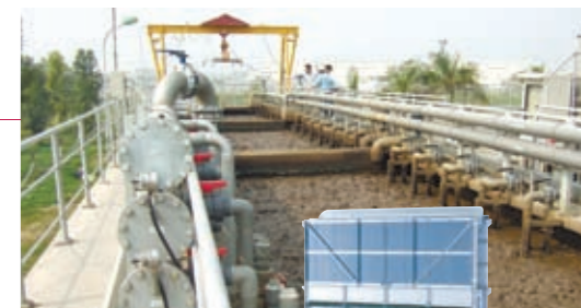
Wastewater treatment facilities in operation
