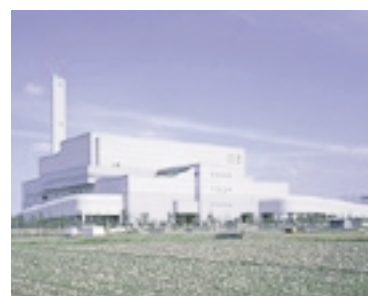
Clean Center East Plant No. 2, Sakai City (460 t/day)
