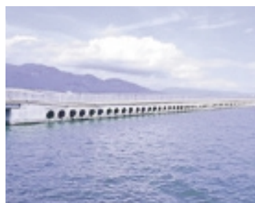
Kubota pipe-style breakwater seepage wall
