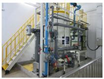
At Kubota Agricultural Machinery (Suzhou) Co., Ltd. (China), we installed recycling treatment equipmen for reusing wastewater from processes throughout the entire plant, and this has realized zero emissions of process wastewater
