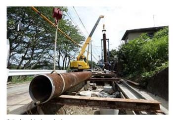
Spiral welded steel pipes
