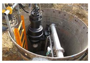
Manhole pumps (for pneumatic transportation of sewage)
