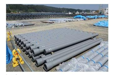
This is used in the restoration and maintenance of lifelines, such as water supplies, sewage lines, and gas lines.
