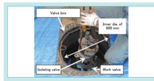
Fig. 11 Replacement Work Inside Valve Box
