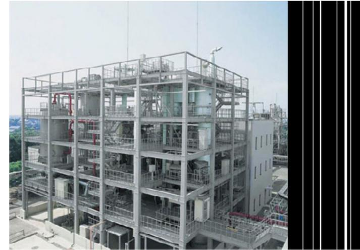
Circulating fluidized bed incinerator (Incinerator No. 2)
