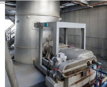
Dewatered sludge (in the form of dewatered cakes) is fed here. 2.5 tons of dewatered sludge per hour is inserted into the continuous type incinerator
